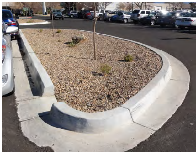
Figure 38: Recently Constructed Parking Lot Island with One Curb Inlet (photo by author)
