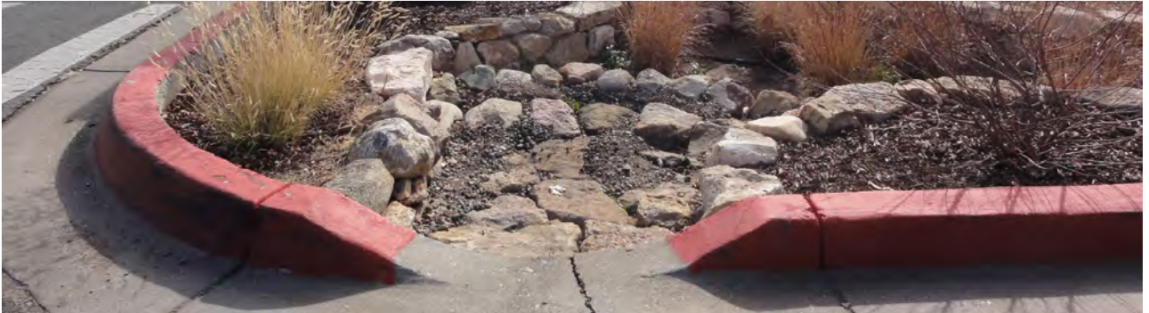
Figure 5: Inlet to Bioinfiltration Basin in the Raincatcher Parking Lot, Santa Fe, NM (photo by author)
