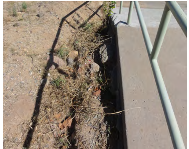
Figure 44: Erosion Undercutting Walkway On Slope (photo by author)
