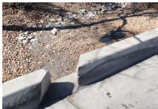
Figure 17: Sediment Accumulation in Infiltration Area, Albuquerque, NM (photo by author)
