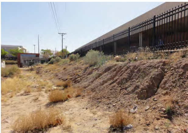
Figure 43: Channels Cutting into Steepest End of Slope (photo by author)
