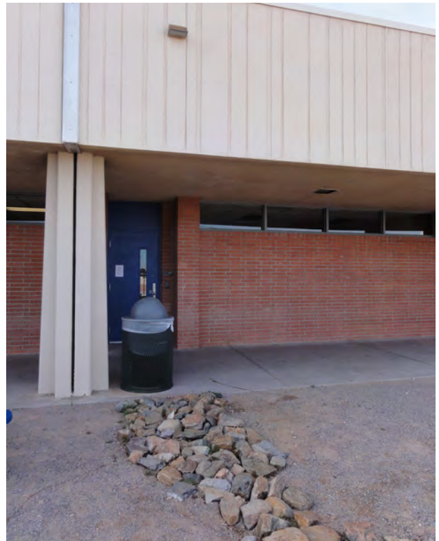
Figure 42: Aggregate Under Canale (photo by author)
