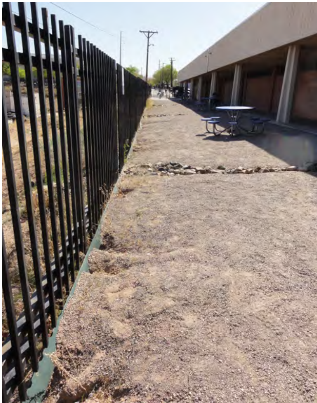
Figure 41: Erosion Along Length of Fence (photo by author)
