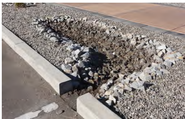
Figure 18: Rock-lined Basin Stained by Runoff After One Year, Albuquerque, NM (photo by author)
